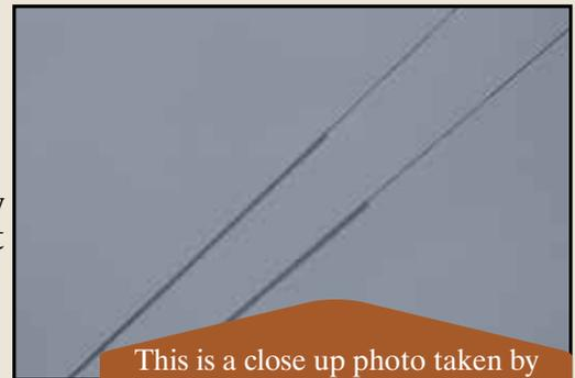
This is a close up photo taken by our crews that shows how snow has the potential to accumulate and weigh down the lines.
