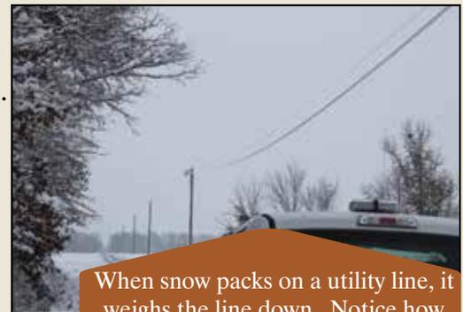
When snow packs on a utility line, it weighs the line down. Notice how the “top” line is sagging below the ground line, causing them to cross.
