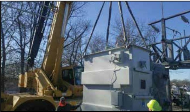
*Reserve substation transformer being moved by crane to its new location.*
